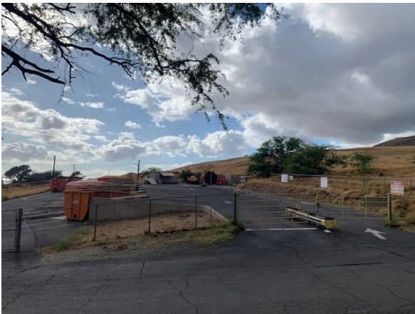
Photo 3: View facing northeast of materials transfer bays and storage containers at Olowalu Recycling Center.
