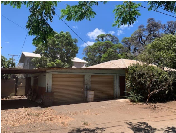
Photo 1: View facing west of 5-gallon and 55-gallon containers located on the east side of property. This was the only publicly accessible viewpoint of the east side of the property.
