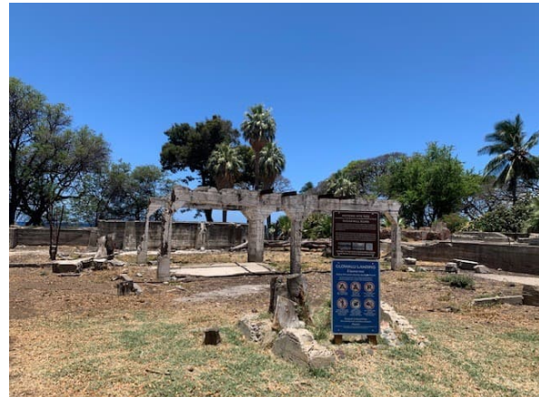
Photo 2: View facing northwest to remaining structures from former Olowalu Company Sugar Mill (EDR Site #3) located at Olowalu Landing.
