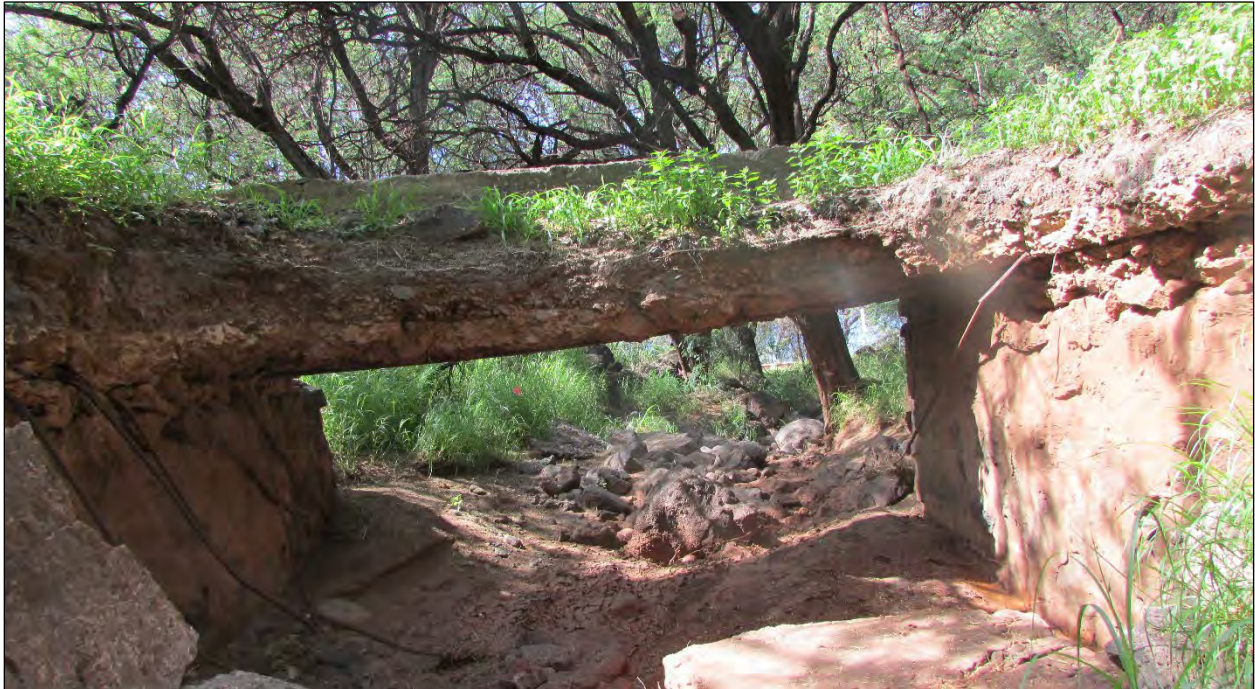
Photo 52. Remnant of an Old Concrete Bridge at the Upper (Eastern) End of the Stream in the Study Area. [Water and sediment staining used to identify the OHWM level here.]
