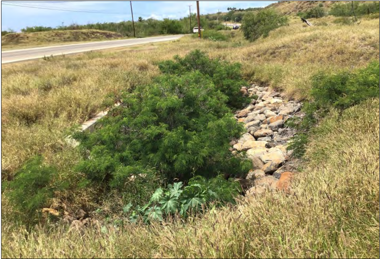
Photo 99. Ka Puali Stream Culvert
