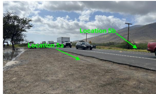
There is no culvert visible on the land side of the existing Honoapiilani Highway at Location 5b in line with Ditch 6.
