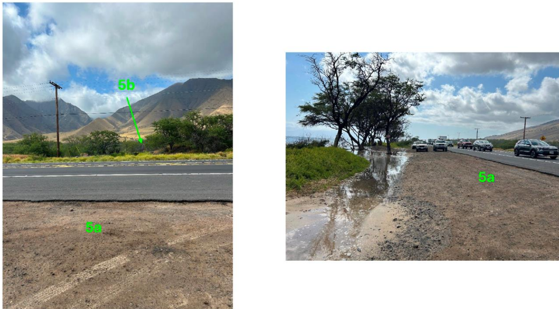
There is no culvert under the existing Honoapiilani Highway at the ocean side at this location
