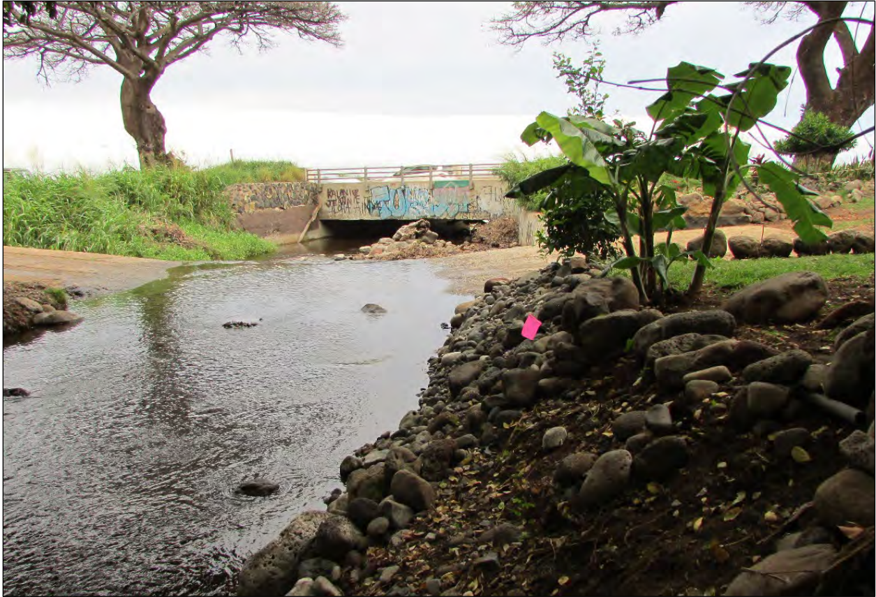
Photo 73. Location of Transect 3 at Lowermost Reach of Stream; Ukumehame Stream Bridge and the Concrete Ford at the Lowermost Reach (The Bridge Footing and Water Staining on the Concrete Defined the OHWM Level for this Lower Reach)
