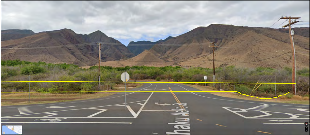
Photo 65. Ditch 8 at Pohaku Aeko Street. [Ditches on Either Side of Pohaku Aeko Street Are Connected Via a Concrete Culvert. Also, the Ditch to the South [Right] of the Road Flows Under the Existing Highway into the Pacific Ocean.]
