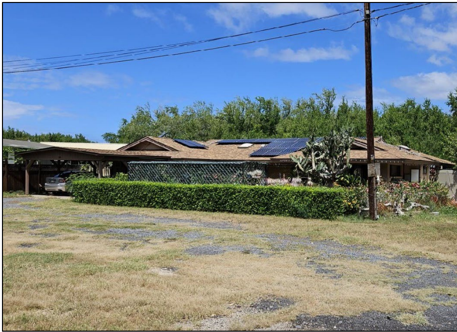
Figure 4.45. Southeast (front) and northeast elevations of AR 11 and outbuilding, facing northwest.
