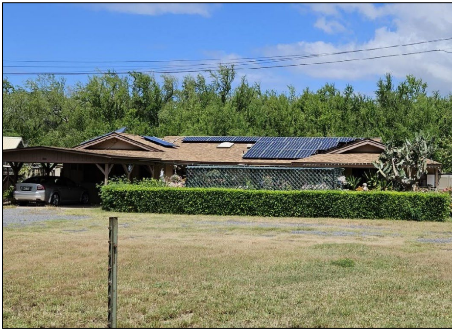
Figure 4.44. Southeast (front) elevation of AR 11, facing northwest.
