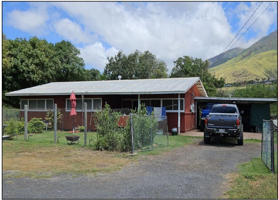
Figure 4.48. South (front) and east elevations of AR 12, facing northwest.
