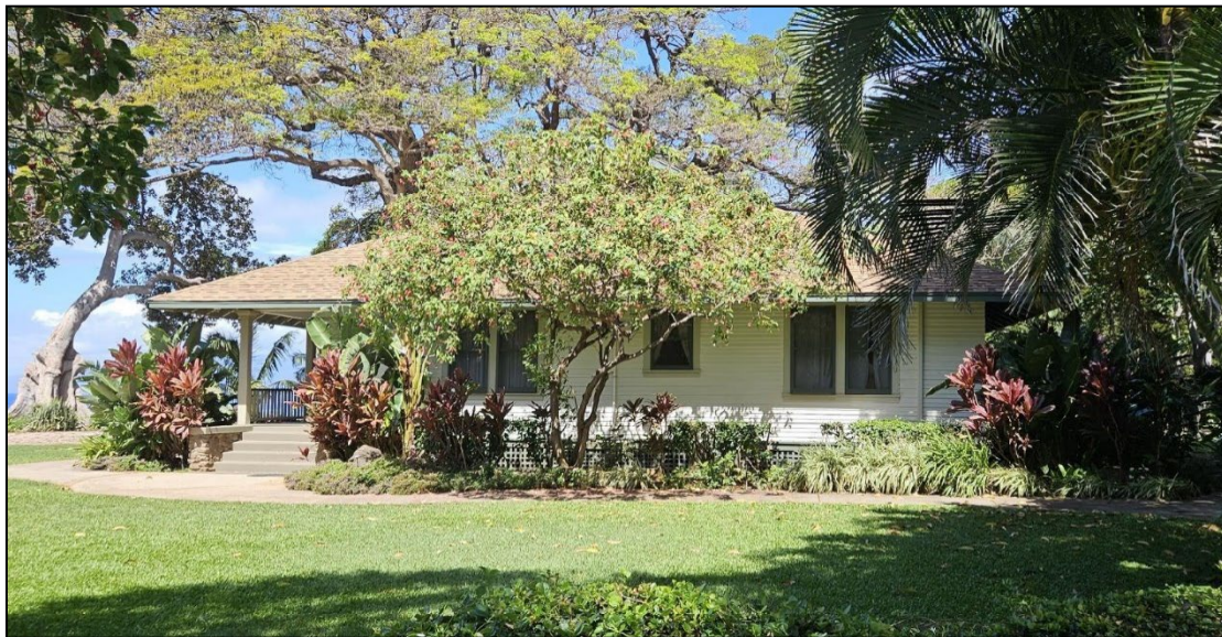
Figure 4.23. East elevation of AR 6, facing northwest.
