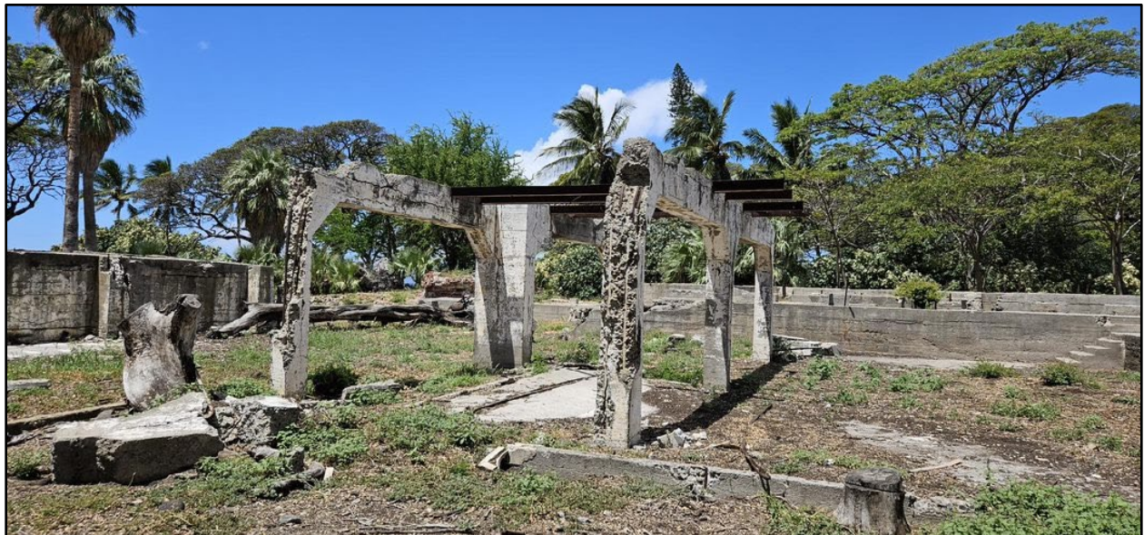
Figure 4.30 . Detail of remnants in area of mud press and centrifugals, facing southwest.
