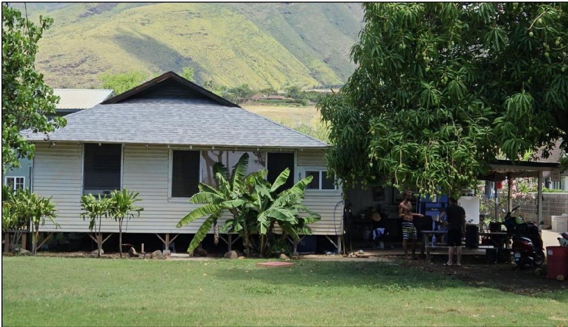
Figure 4.53. South (front) elevation of AR 13, facing northwest.
