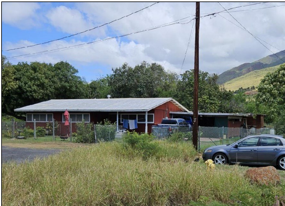
Figure 4.50. South (front) and east elevations of AR 12 and outbuilding, facing northwest; note the outbuilding beyond the carport.
