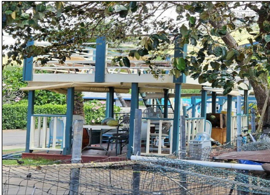
Figure 4.58. View of detached two-story deck, facing northwest.
