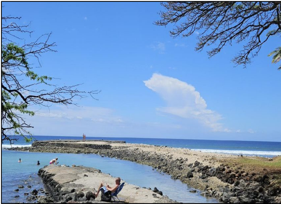
Figure 4.29 . North (front) east and elevations of Olowalu wharf piers, facing southwest.
