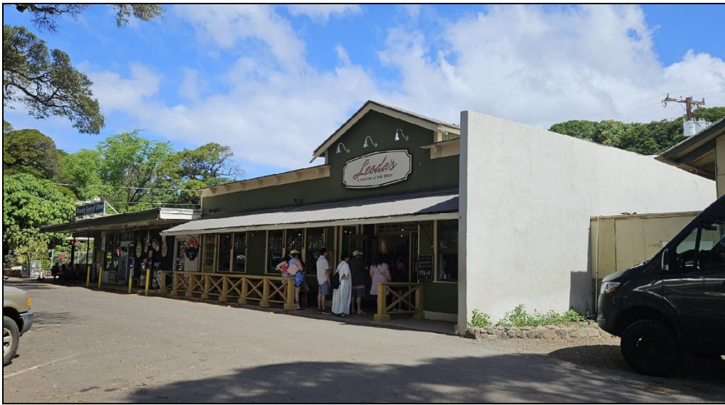
Figure 4.10. South (front) and east elevations of AR 3, facing northwest.
