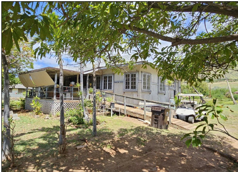
Figure 4.67. South (front) and east elevations of AR 16, facing northwest.
