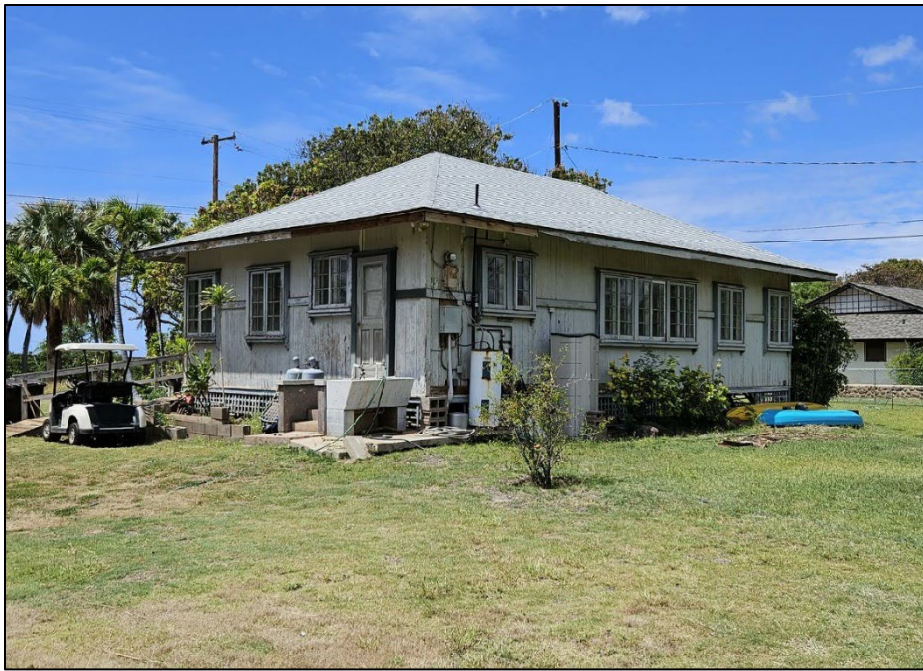
Figure 4.70. South elevation of outbuilding, facing north.
