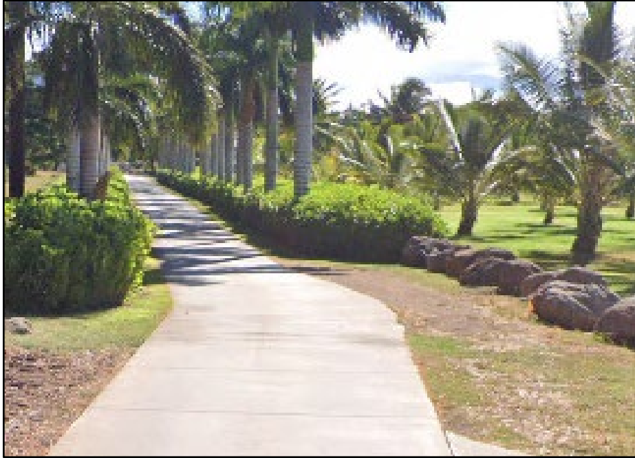
Figure 4.121. View of a portion of AR 26, facing east.
