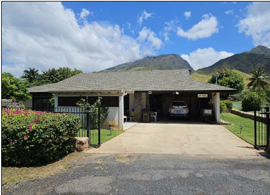
Figure 4.62. South (front) elevation of AR 15, facing north.
