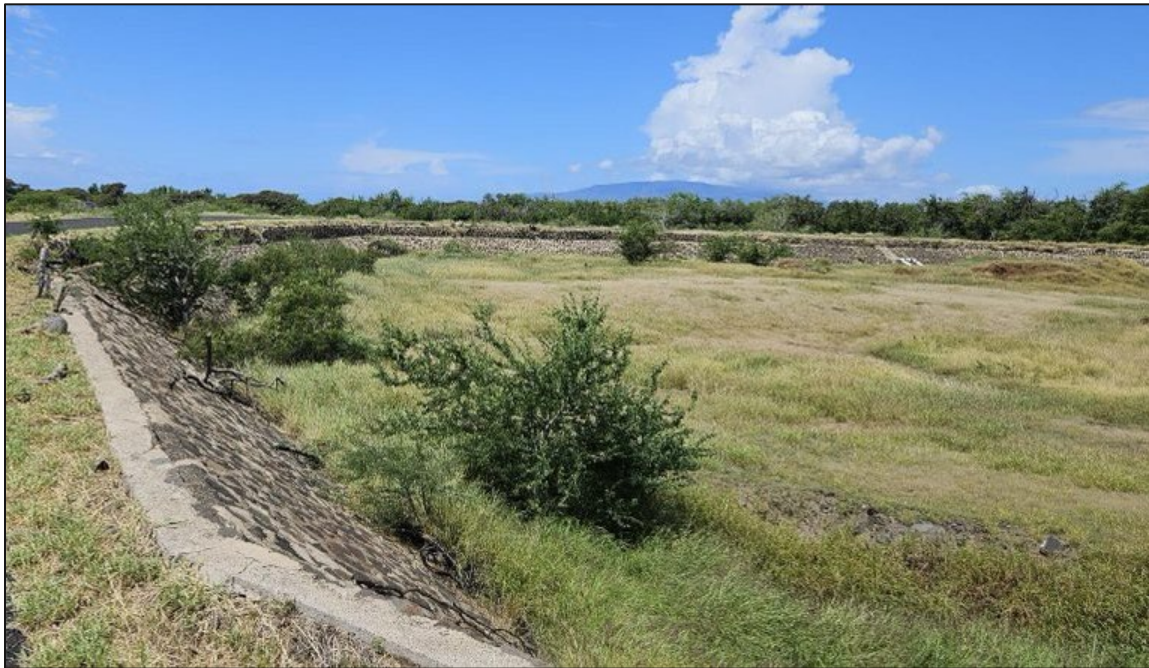
Figure 4.36. Southeast, south, and southwest walls of AR 9, facing south.
