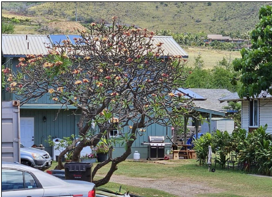
Figure 4.55. South elevation of outbuilding, facing north.
