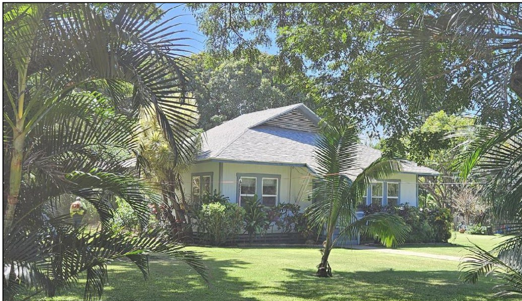
Figure 4.17. North and west (front) elevations of AR 4, facing southeast.
