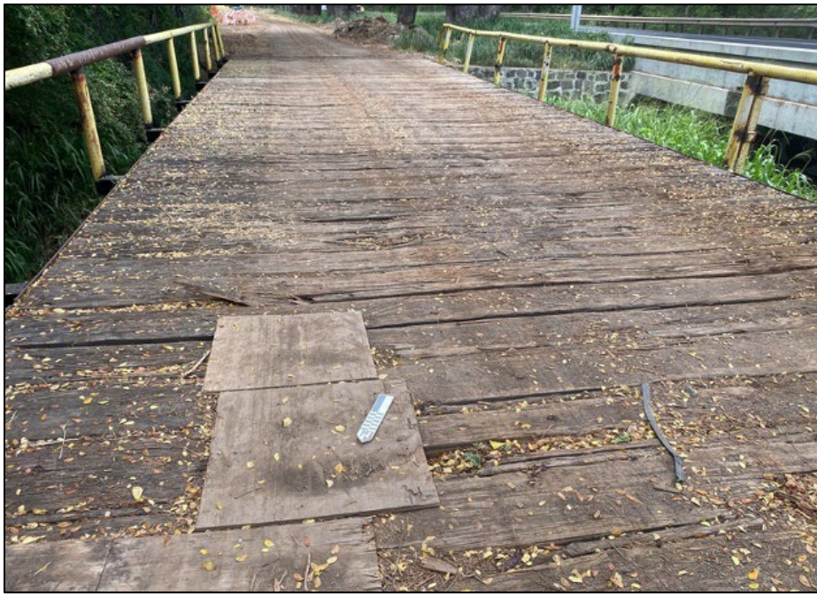
Figure 4.89. Detail of AR 20 wood deck boards and plywood repairs, facing southeast.
