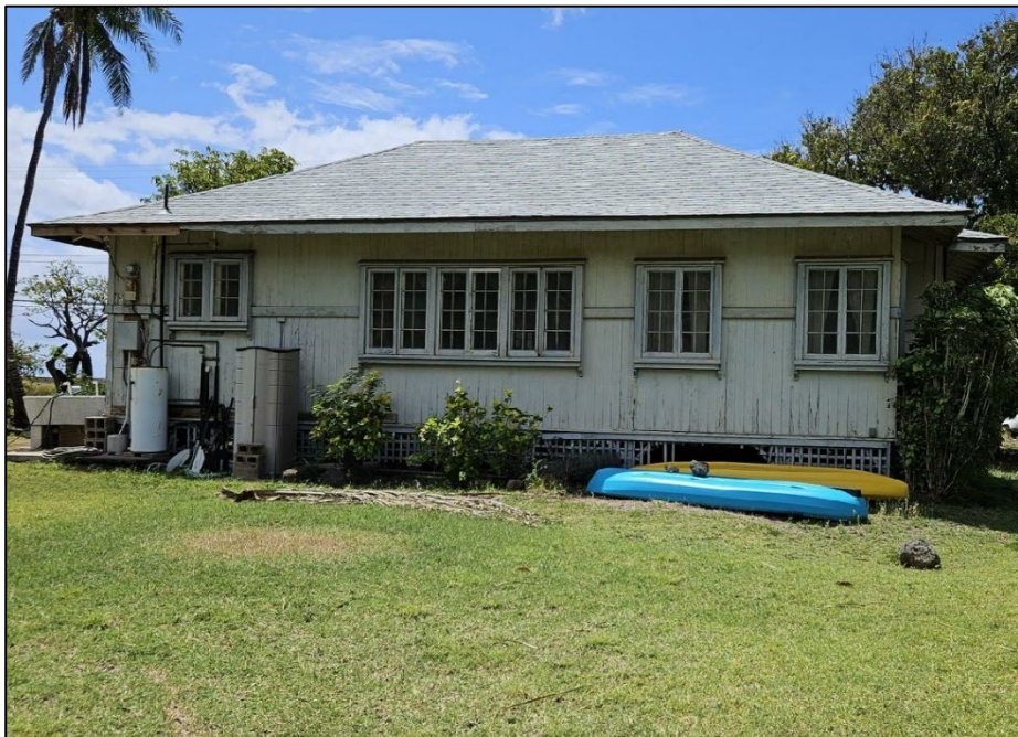
Figure 4.69. North (rear) elevation of AR 16, facing south.
