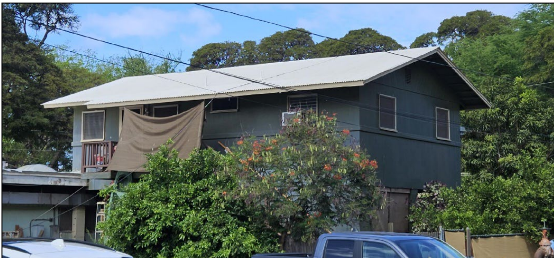
Figure 4.13. East and north (rear) elevations of the second addition of AR 3, facing west-southwest.
