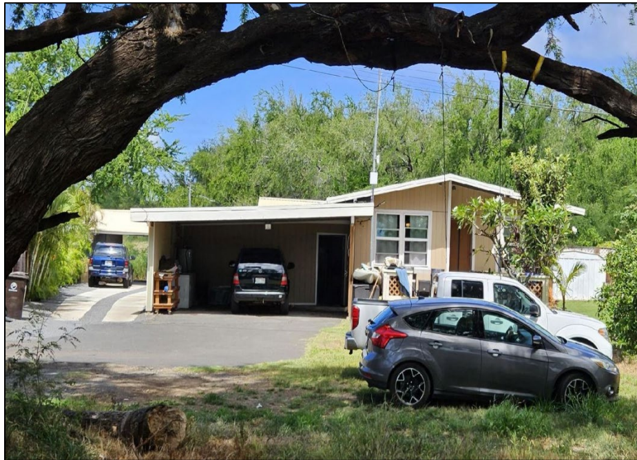
Figure 4.40. Southeast (front) elevation of AR 10, facing northwest.
