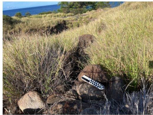
Plate 91. Overview of west extent where the barbed fence component bisects wall, view to west.
