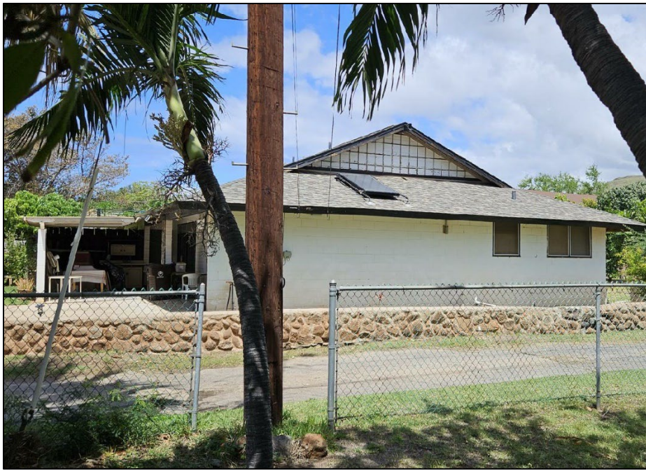
Figure 4.63. East elevation of AR 15, facing west.
