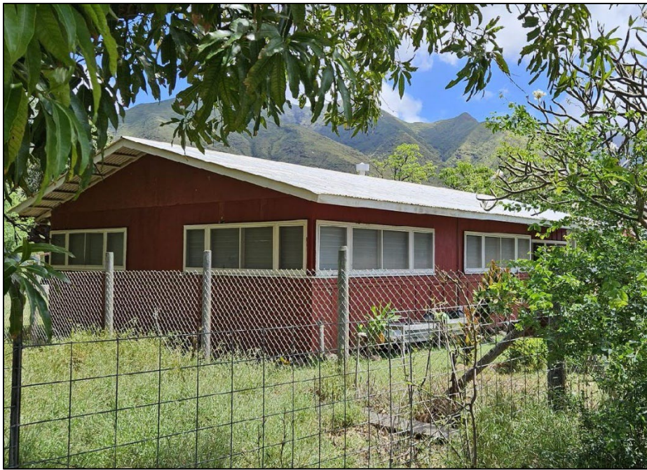
Figure 4.49. South (front) and west elevations of AR 12 and outbuilding, facing northeast.
