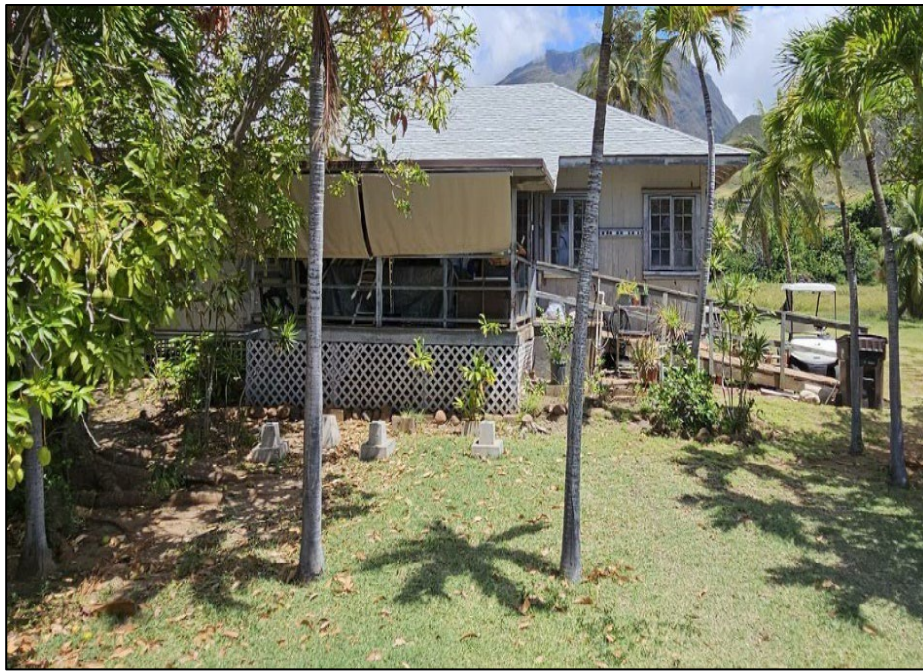
Figure 4.66. South (front) elevation of AR 16, facing north.
