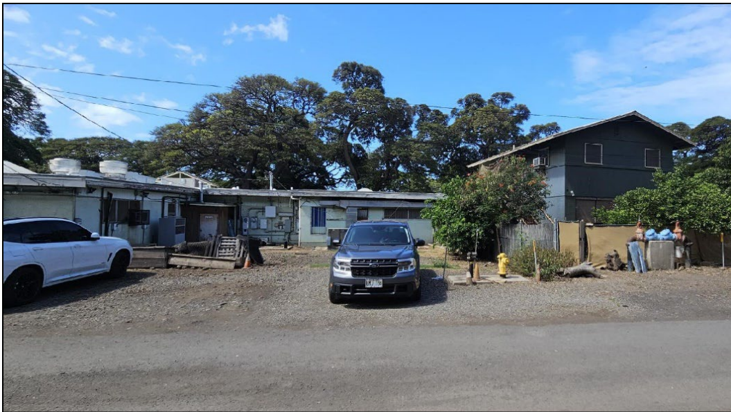
Figure 4.12. North (rear) elevation of AR 3, facing west-southwest.
