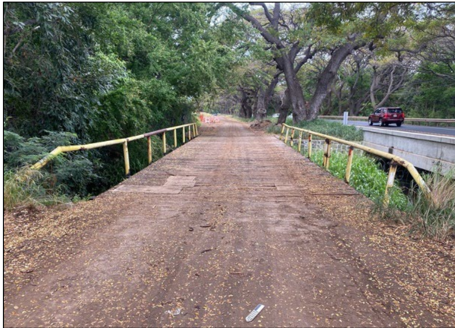
Figure 4.88. Deck and west elevation of AR 20, facing southeast.
