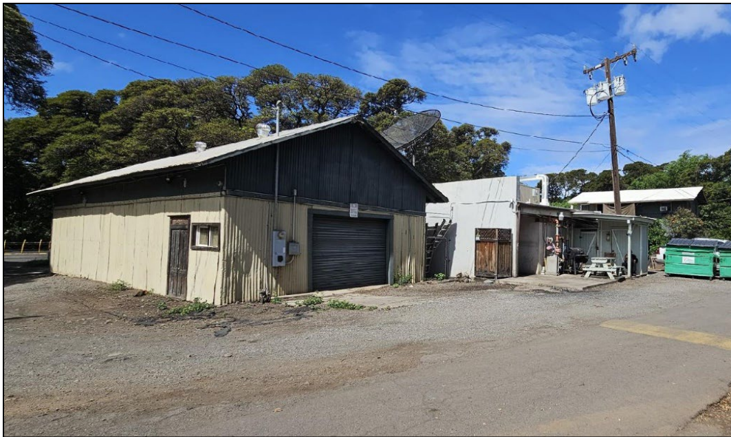
Figure 4.14. East and north (rear) elevations of AR 3, facing southwest.
