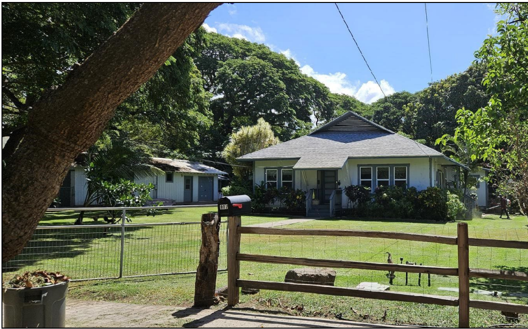
Figure 4.16. West (front) and south elevations of AR 4, facing east.
