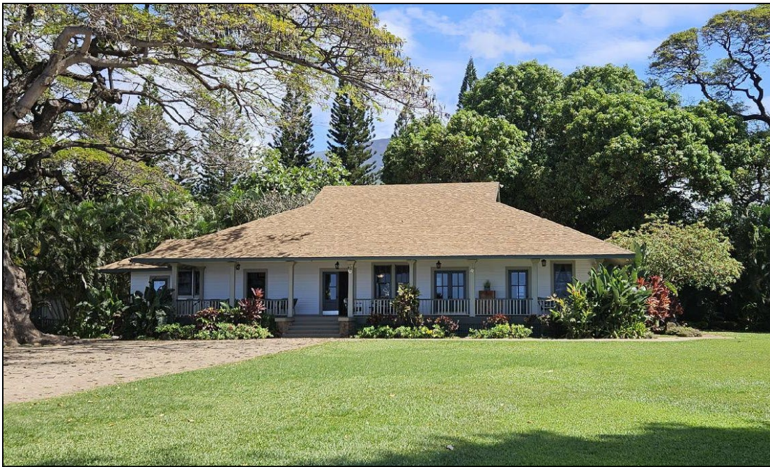
Figure 4.22. South (front) elevation of AR 6, facing northeast.
