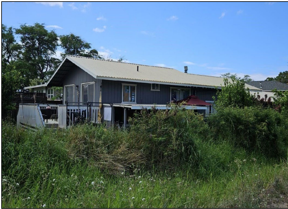
Figure 4.41. Northeast elevation of AR 10 and outbuilding, facing south.
