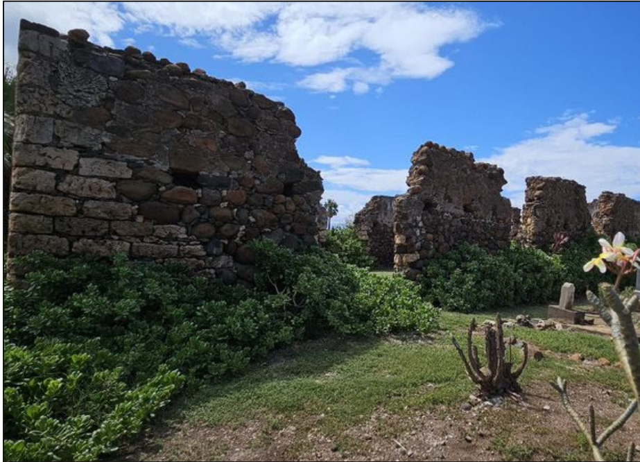
Figure 4.76. West elevation of stone church, facing southeast.
