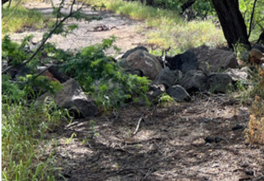
Figure 4.133. Image of the character and condition of AR-29, an exceedingly common Plantation era concrete and stone infrastructure found in the region.
