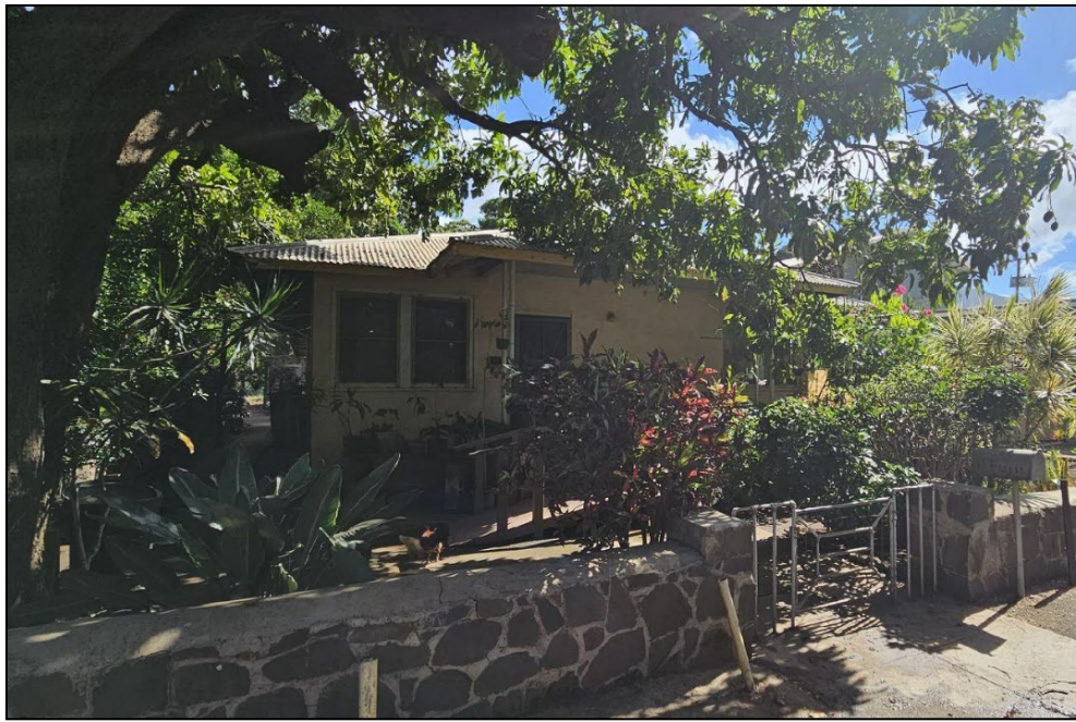
Figure 4.7. South (front) elevation of AR 2, facing northeast.
