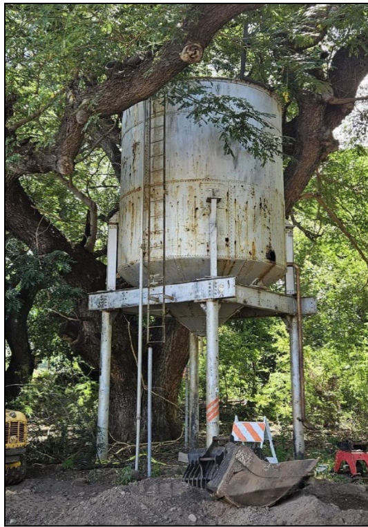
Figure 4.85. Water tower associated with AR 19, facing northeast.
