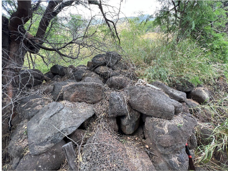
Figure 30. AA2226-097, section of wall showing intact facing, as well as, a section affected by vegetation growth, view to northeast.
