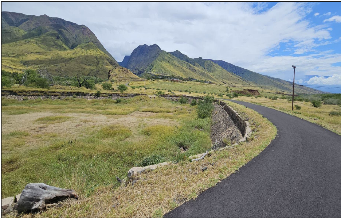
Figure 4.37. Modern impact from the construction of a bike path along the south and east elevation of AR 9, facing east.
