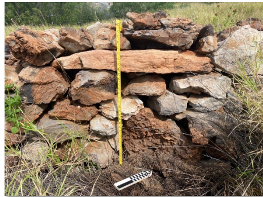
Plate 113. SIHP 50-50-08-05954, close-up of wall face, view to northwest.
