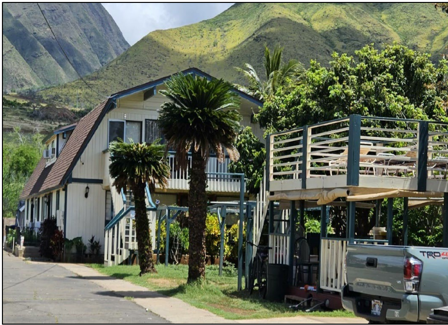
Figure 4.59. South and east elevations of AR 14, facing north.
