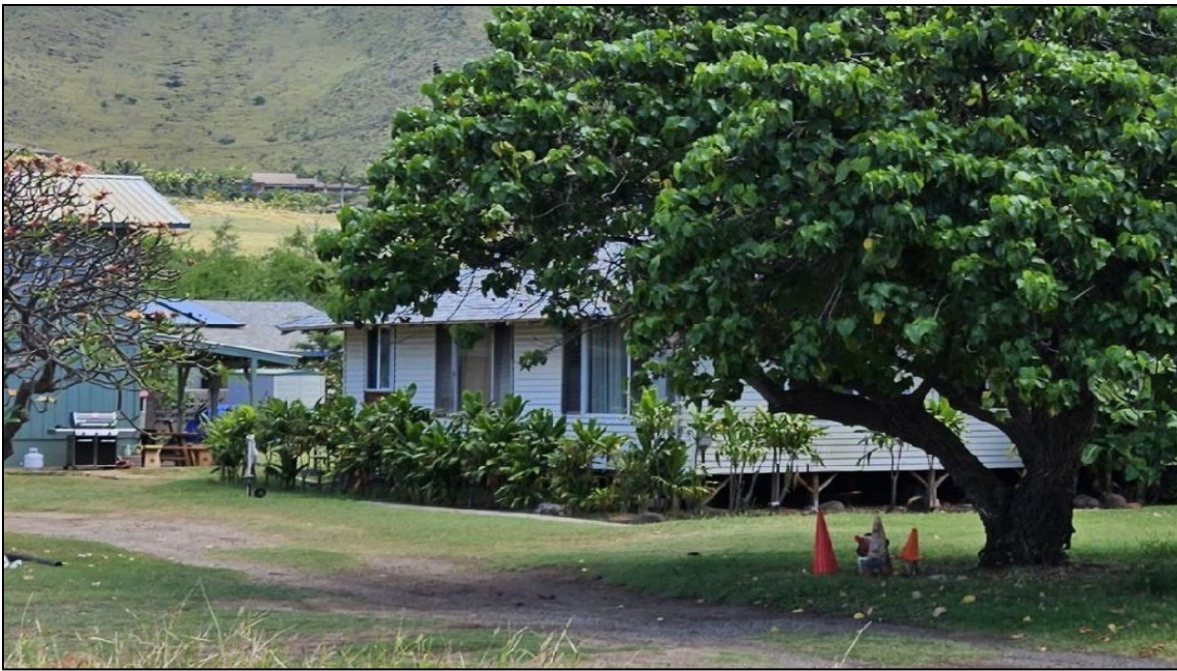
Figure 4.54. South (front) and west elevations of AR 13 and outbuilding, facing northwest.
